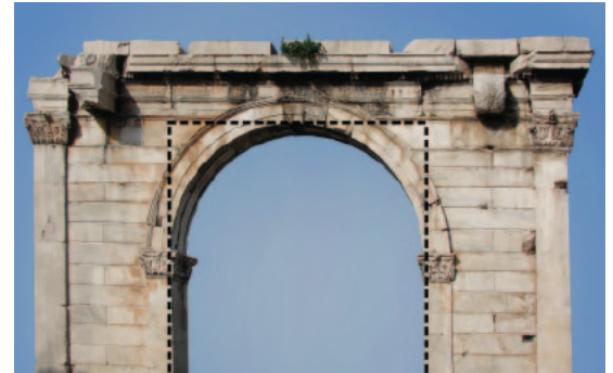
Wall whose area is calculated as if its opening were along the dotted lines
