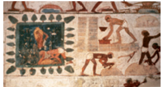
The manufacture and transportation of bricks, Tomb of Rekhmire, 15th century BCE
